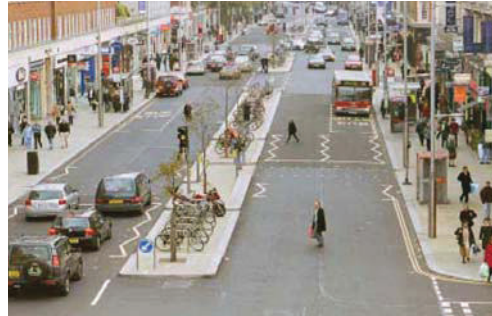
Above: High Street Kensington, London. Example of de-cluttering, removal of obstacles to pedestrian movement, cycle parking provision etc. Recorded accidents have been considerably reduced following implementation.
