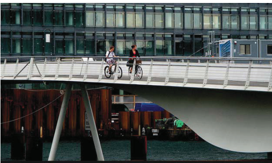
Above: Cycle and foot bridge, Copenhagen, Denmark
